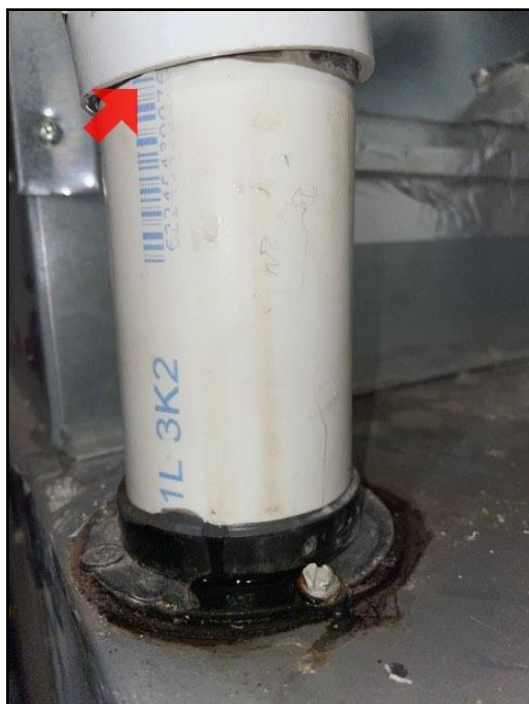
Poor connections
