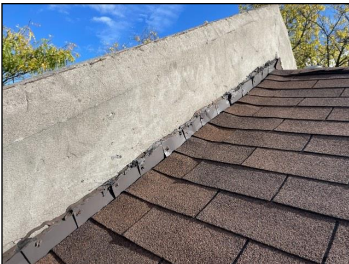
Counterflashing missing
